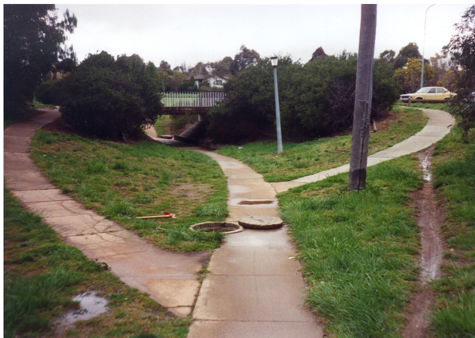
Figure 5.3.6 Manhole Entry to 300 mm diameter Pipe Gauge
