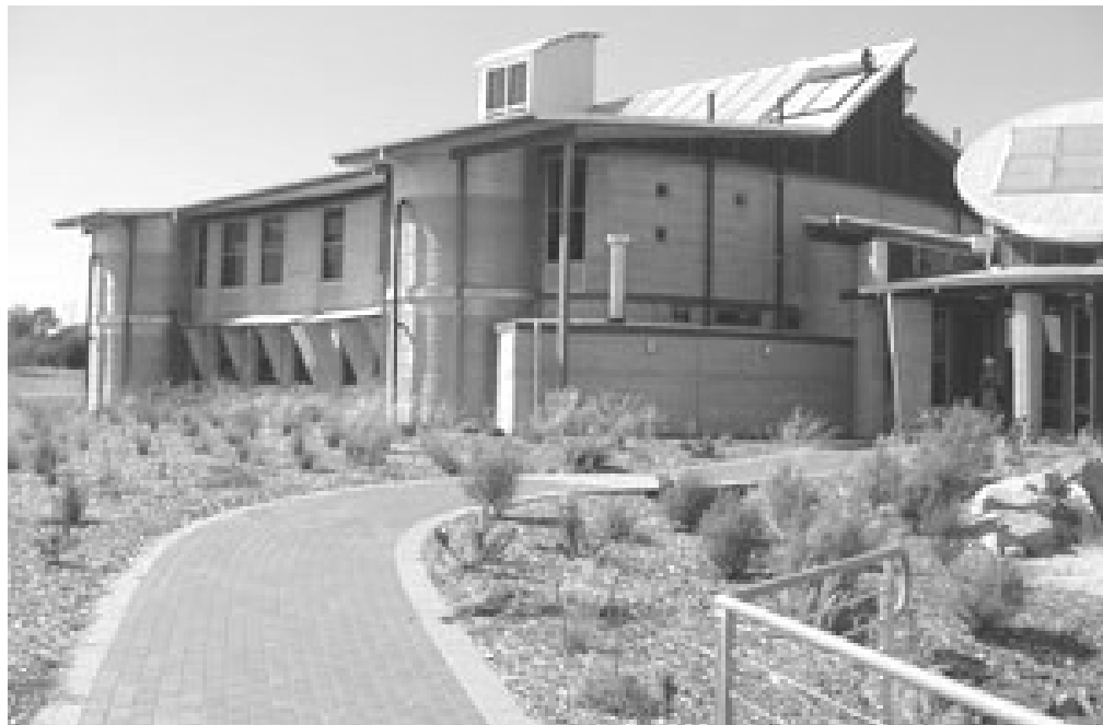
Figure 1.7 Stabilised Rammed Earth Building at Albury, NSW
