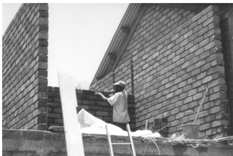
Figure 1.6 - Pressed Earth Brick Building under Construction in Mayotte
