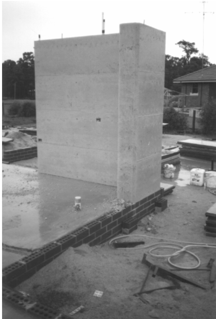
Figure 1.3 Rammed Earth House under Construction (Margaret River)
