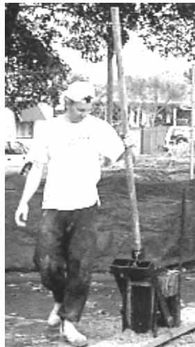
Figure 1.4 - Making Pressed Earth Bricks using “Cinva Ram” Type Machine
