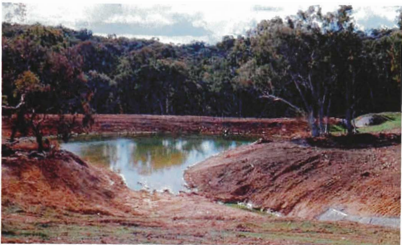
Figure 4.8 Runoff collection dam at the base of the barren slope after remediation. Viewed towards the west.
