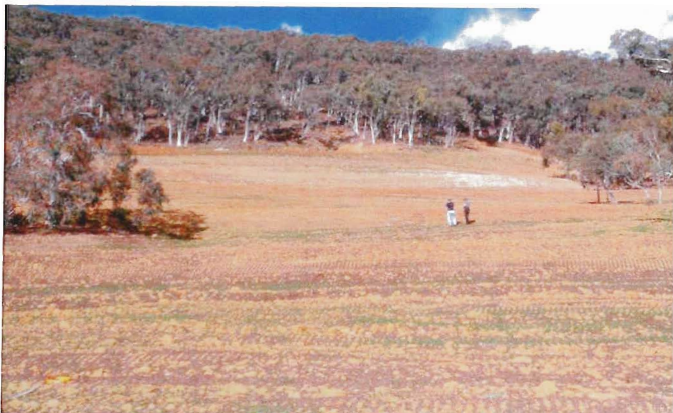
Figure 4.9 The barren slope after the second remediation attempt. Brown soil colouration in the foreground is biosolid. Light green cereal pasture mix was used for site stabilization. The chalk-coloured surface behind the figures is the acid seep. The “lone gum” (See Fig. 3.1) is present in the centre-left of the slope. Viewed towards the northeast.
