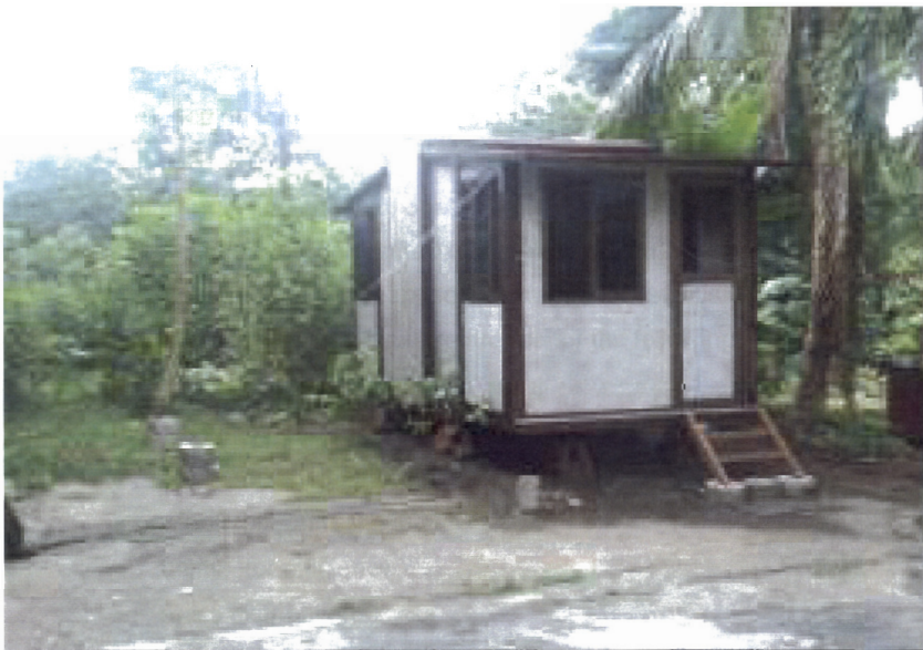
Figure 2.5. The lumber-framed shop-fabricated emergency shelter, complete with false posts (used to cover of the wall to wall connection), stairs and tie-down straps anchored to ground, currently being service tested at the FPRDI.
