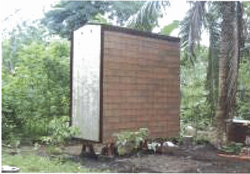
Figure 2.2. The emergency shelter is delivered to the site in a rigid case. The rigid case is mounted on adjustable prefabricated footings
