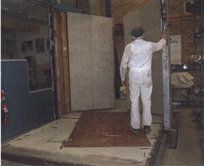
Figure 6.3 Side walls 2 and 6 were erected.
