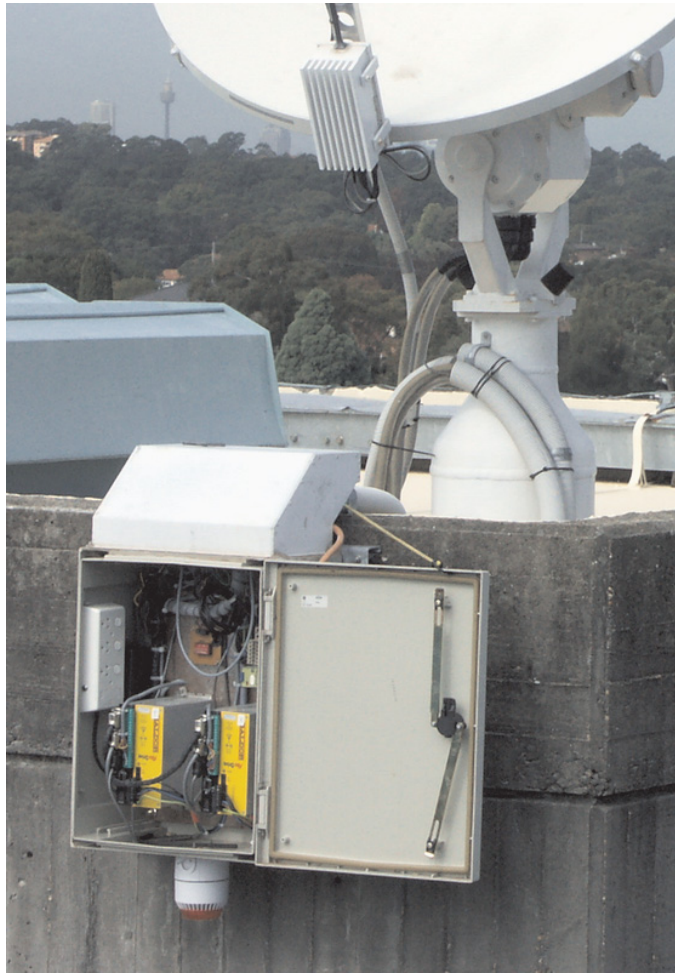
Figure 4.8: Outdoor unit with drive enclosure and pedestal
