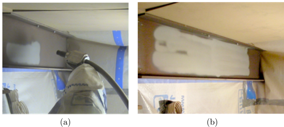
FIGURE 6.30: A manipulator conducting grit-blasting of a metal I-beam surface based on a map autonomously generated by AXBAM.
