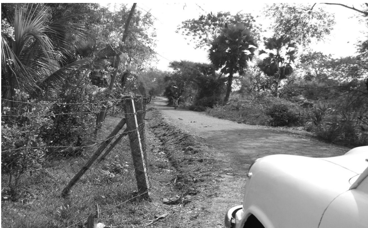
D.4: The brick-built road made by the villagers – the only connection to the city - BAS
