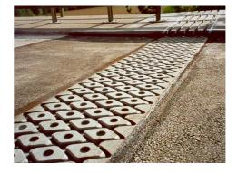
**Figure 2.3(b)** Welded rhombic plates (Courtesy Maurer-Söhne GmbH)
