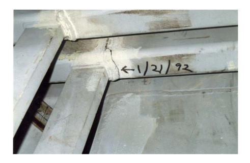
**Figure 3.2** Centre beam cracking – 3<sup>rd</sup> Lake Washington Bridge After Roeder (2004)
