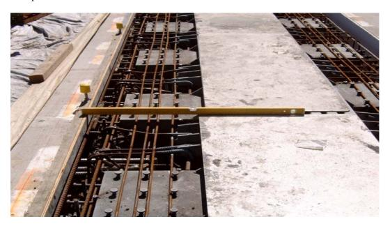
**Figure 2.6** Karuah MBEJ during installation
