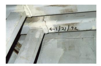
Figure 3 Centre Beam Cracking – 3<sup>rd</sup> Lake Washington Bridge (After [14])
