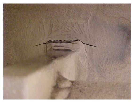
Figure 3 Typical Cracking above Asymmetric Internal Stiffener
