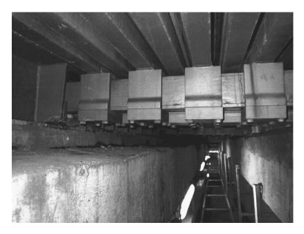
Fig. 2. View of Anzac Bridge MBEJ, western abutment
