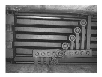
Fig. 3. View of underside of Anzac Bridge modular joint
