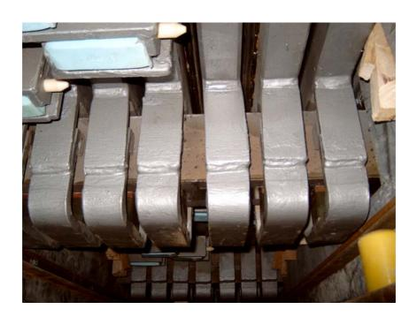
**Figure 1.3** Example of a single support bar MBEJ design
