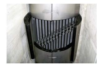
**Figure 2.2(a)** Partially encapsulated joint – Itztal Bridge (Germany)
