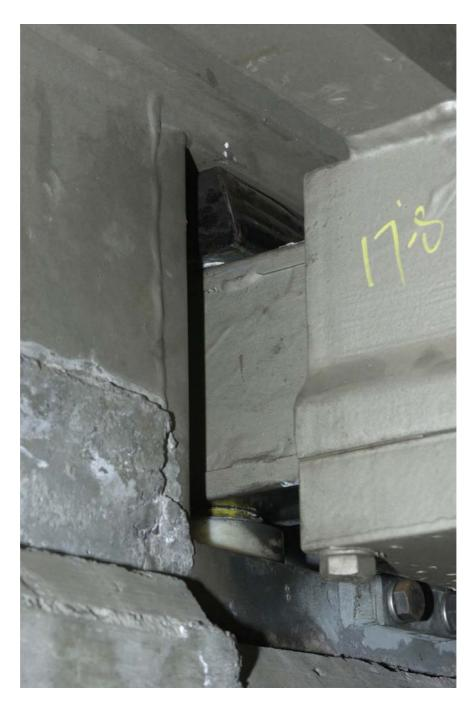
Figure 3.12 Distorted upper support bar bearing
