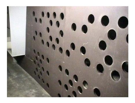
Figure 2.1 Helmholtz absorber installation at Tom Ugly's Bridge
