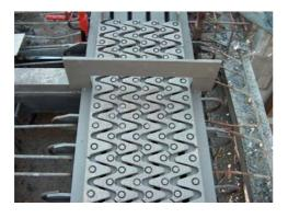
**Figure 2.3(a)** Bolted sinus plates (Courtesy Mageba SA)
