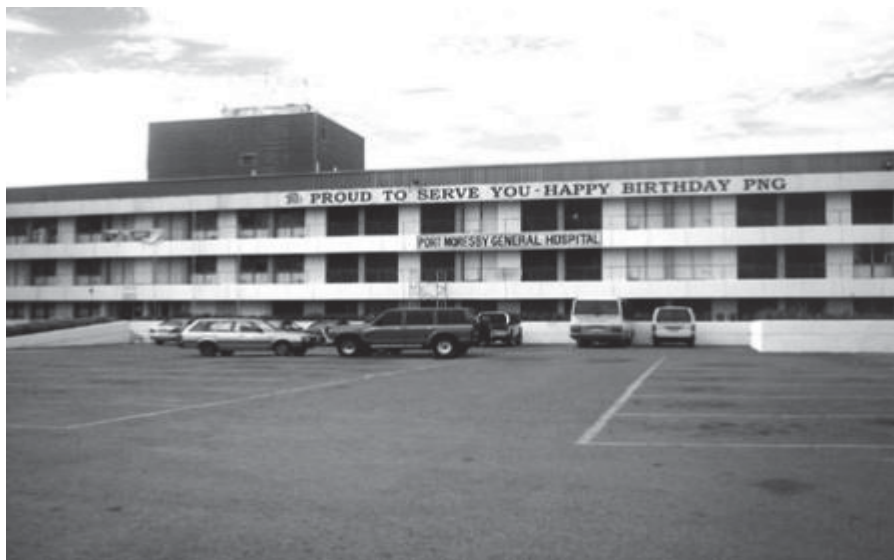
Figure 1: Port Moresby General Hospital front block built by the Australian Government in 1974
