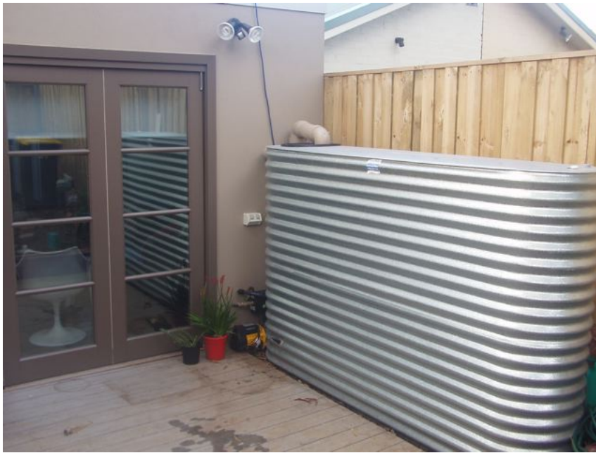
Figure 5-4 Example of a domestic rainwater storage tank
