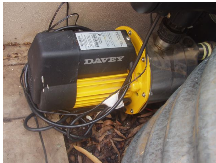
Figure 5-5 Example of a domestic rainwater pump
