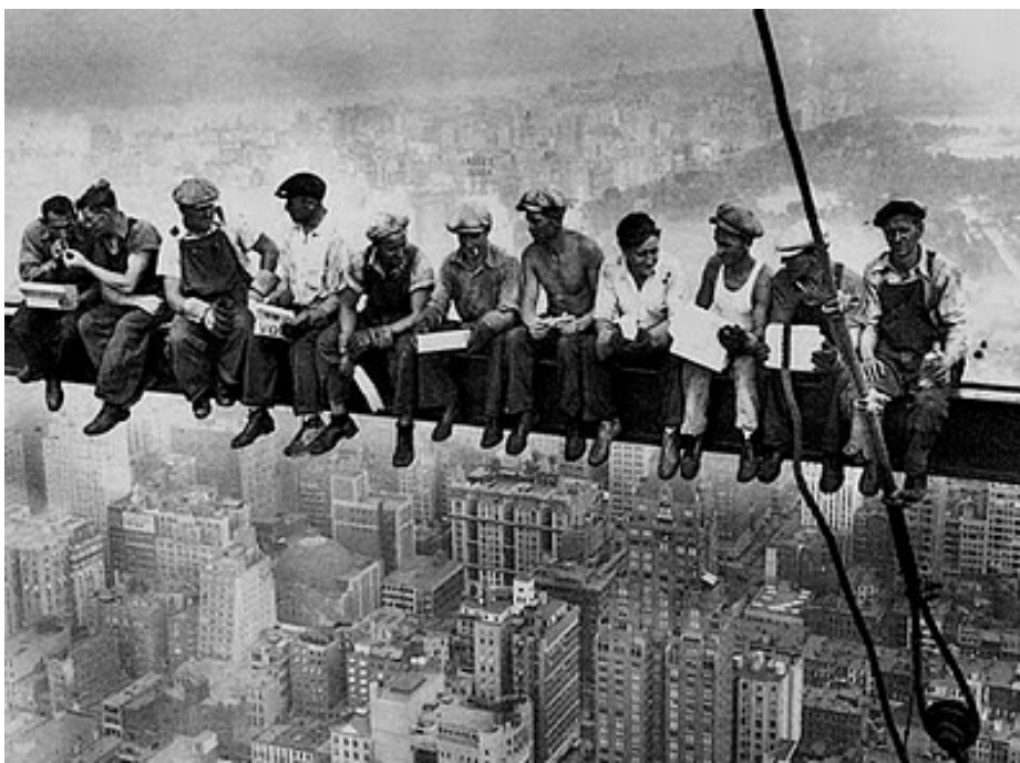
Figure 38B: Empire State Construction Workers. Photo: Lewis Hine, c.1931
