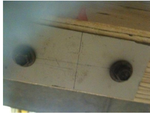
(a) Metal plate on concrete topping (b) Metal plate on LVL timber joist
