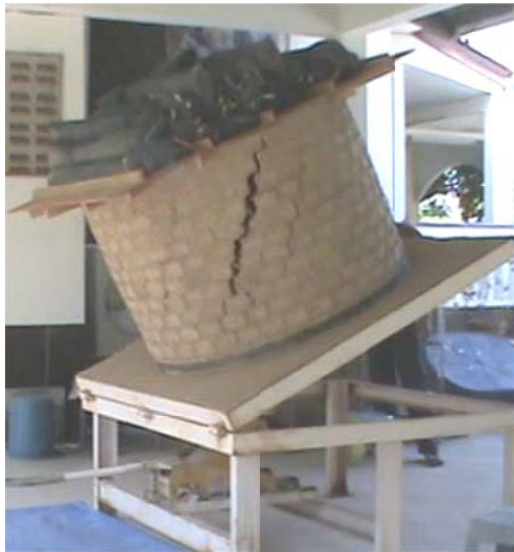
(3)Another crack appeared.
