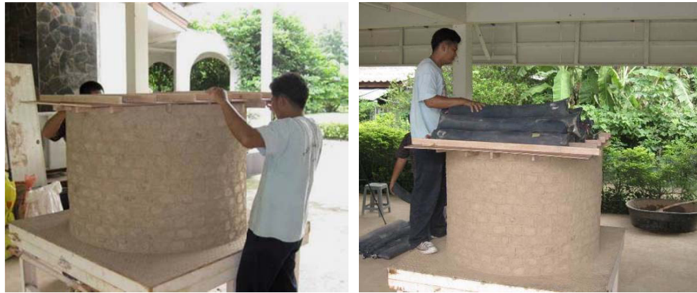
Figure 8.5: Roof and sand bags installation.
