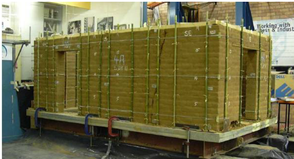
Figure 2.18: Damaged model adobe house retrofitted with string, bamboo, wire and timber ring beam at UTS (Dowling 2006).
