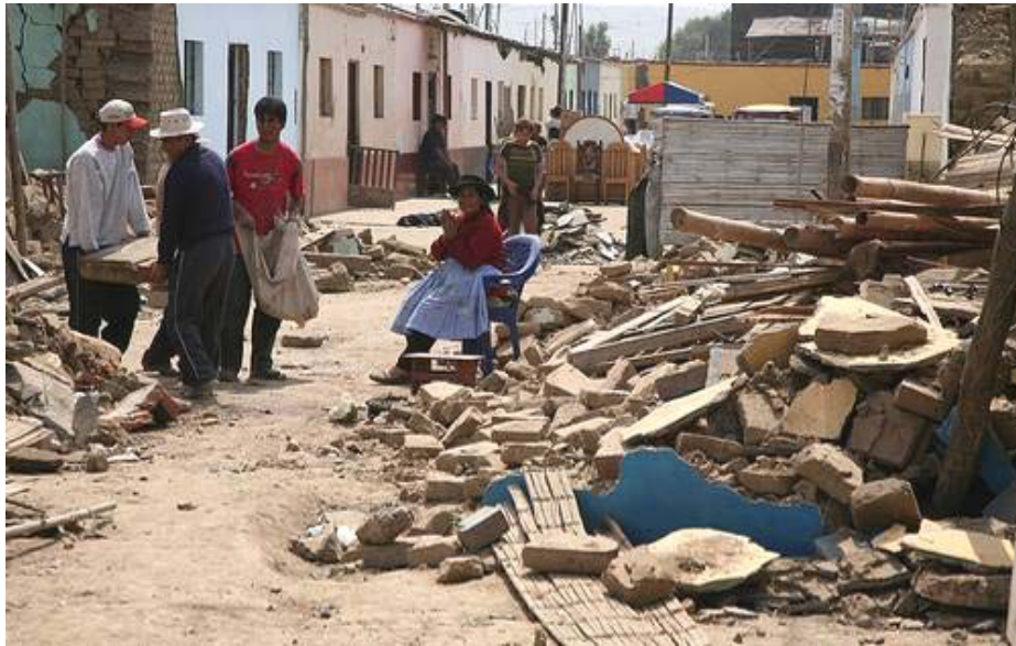
Figure 1.7: Earthquake damage to adobe houses Peru-Aug 16, 2007 (Jean Luis Arce /Reuters).
