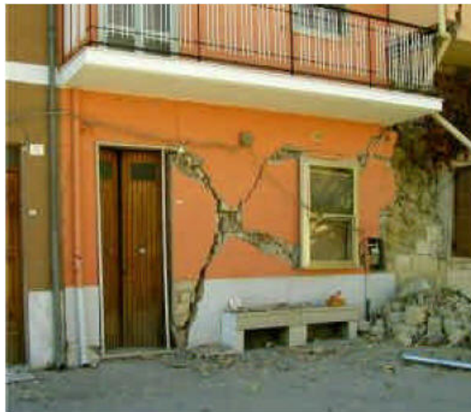
Figure 3.9: In-plane shear failure – San Giuliano (Marrow).
