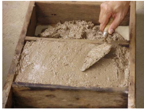
(b) Mud was placed into mould
