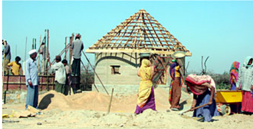
Figure 1.10: The quake-safe circular Adobe houses in India.(swissinfo.ch).
