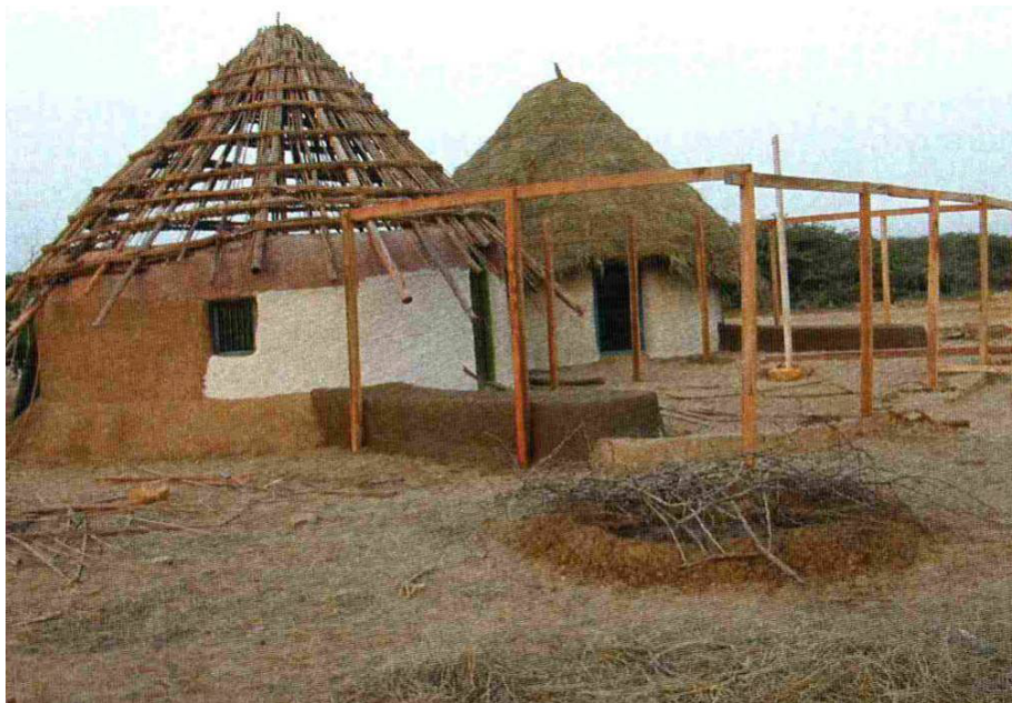
Figure 4.15: Typical circular earthen hut of Kutch district (Amir January 2005).
