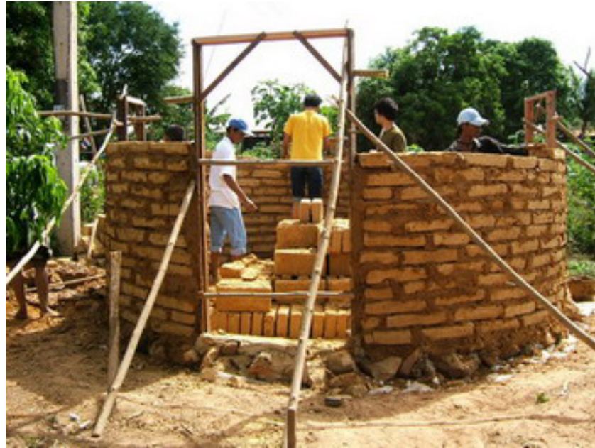
Figure 7.11: Circular-adobe-wall construction.
