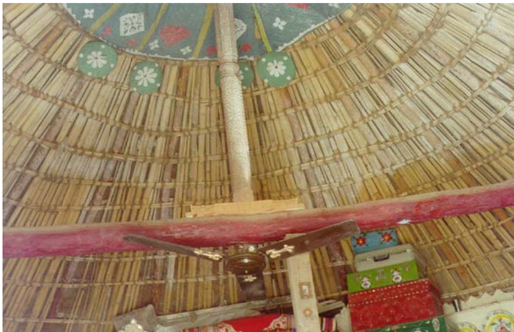
Figure 4.18: Light roof structure of Bhunga house.
