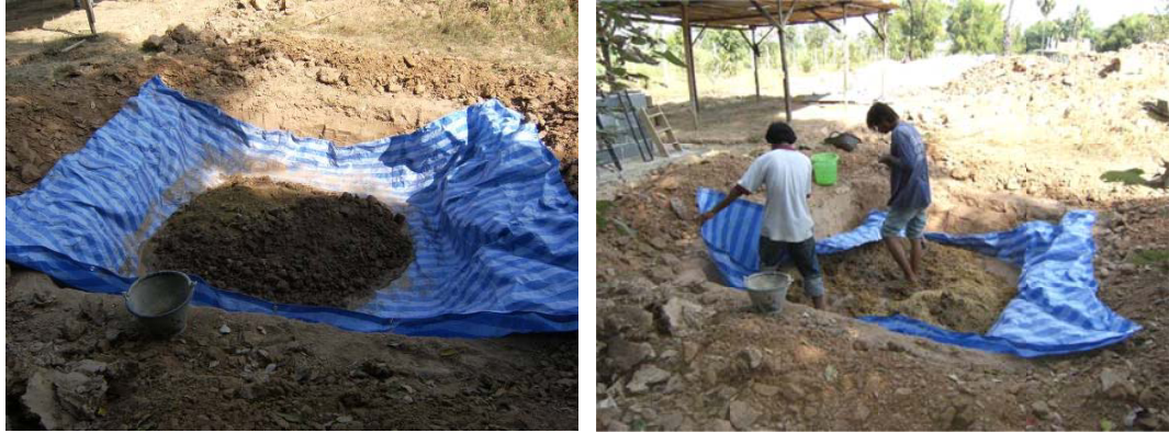
Figure 6.1: Mixing of mud for adobe bricks.
