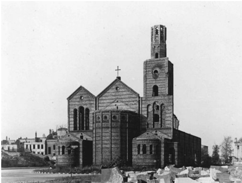
32. St Matthew's Church ruins northern side (1952)
