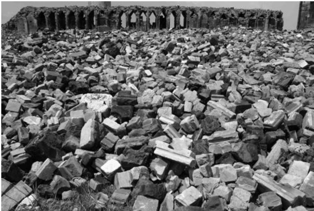
19. Processing plant under demolition, Chicago (2009)
