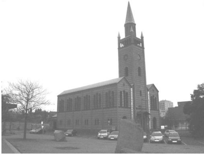
33. St Matthew's Church southern side (2011)
