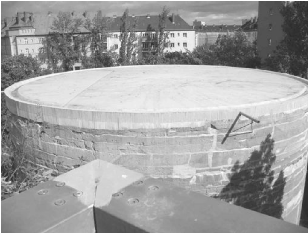
43. The top of the Schwerbelastungskörper from the viewing platform (2011)
