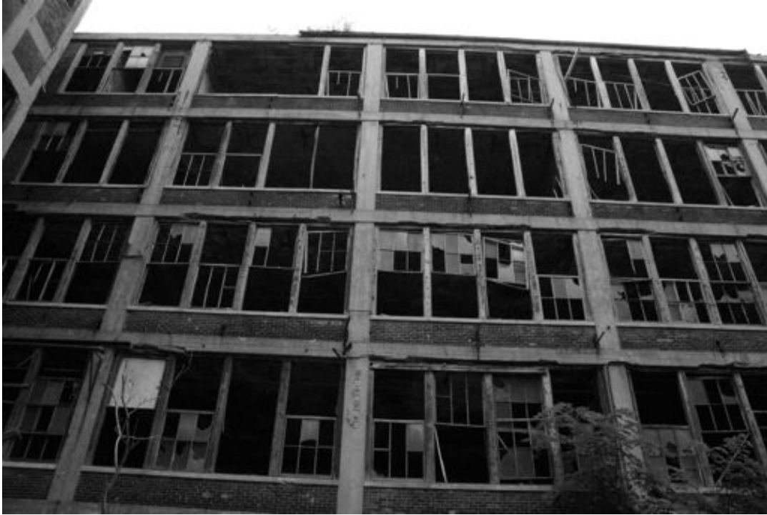
53. Packard Plant windows (2009)
