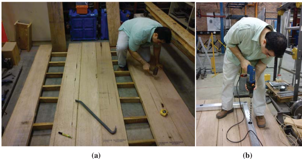
Figure 4.17: (a) Construction of timber base plate at the structures laboratory; (b) drilling required holes on the timber base plate
