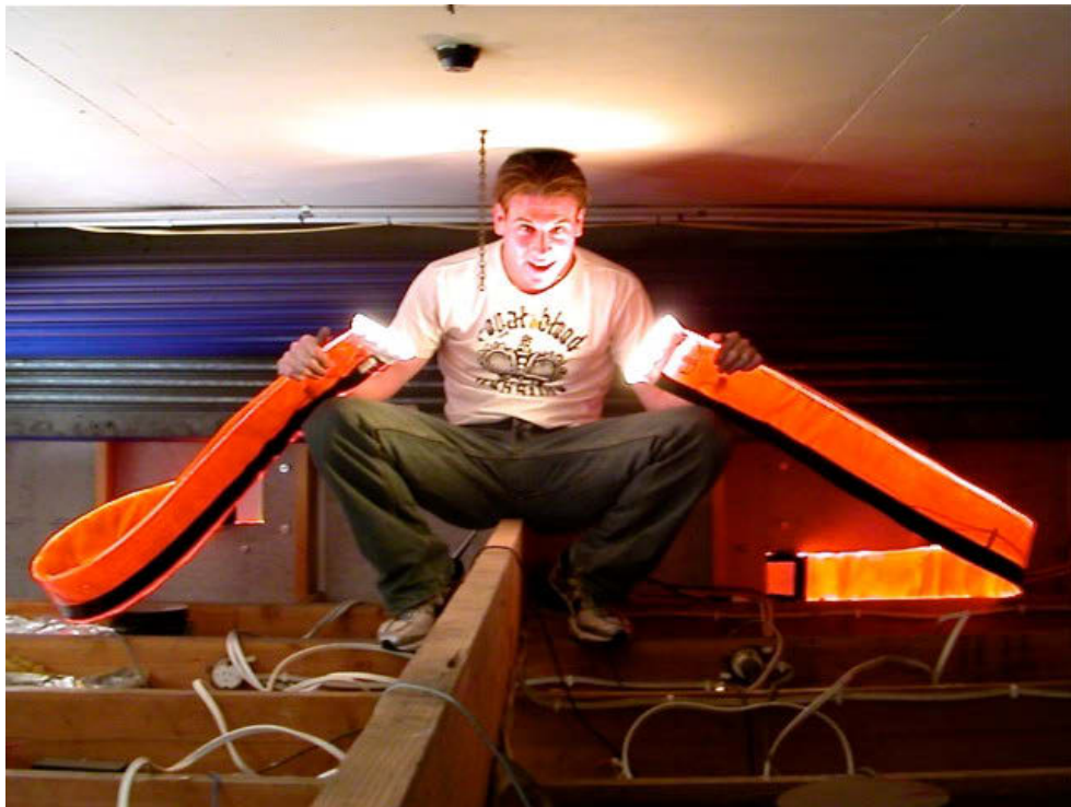
Figure 3.26 Installation of the hybrid SCATS system.
