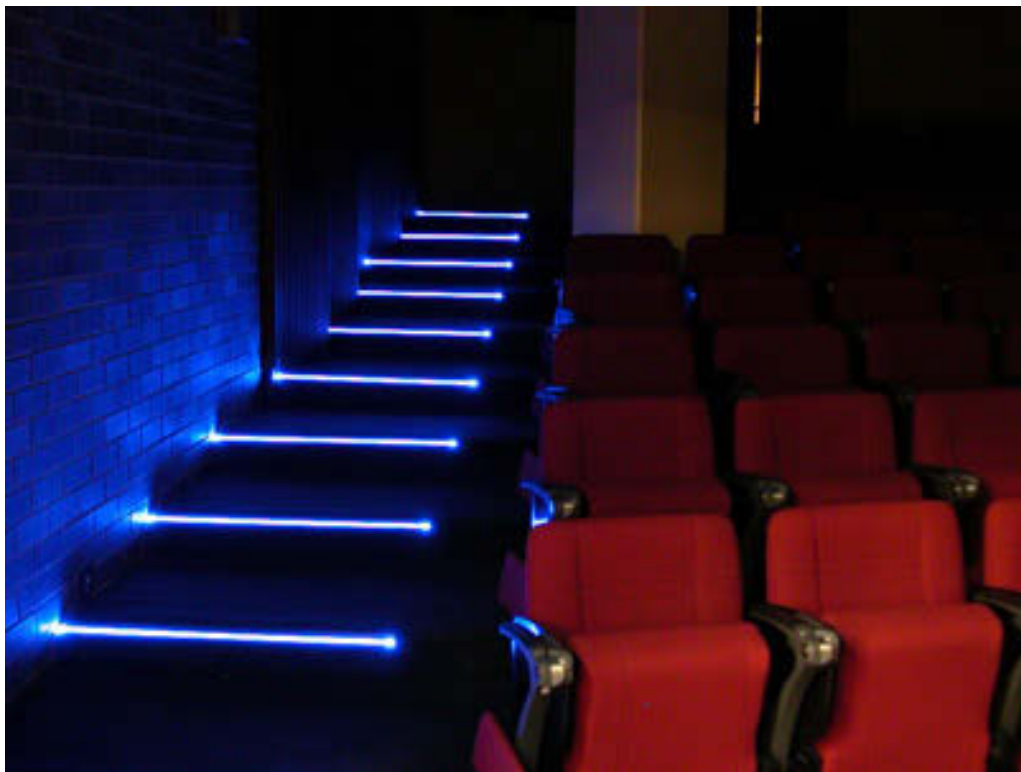
Figure 5.17 Stair lights at UTS using TRIMM doped side-scattering optical fibre.
