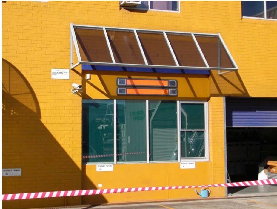
Figure 3.25 Façade mounting of two hybrid SCATS collectors to illuminate an interior room.
