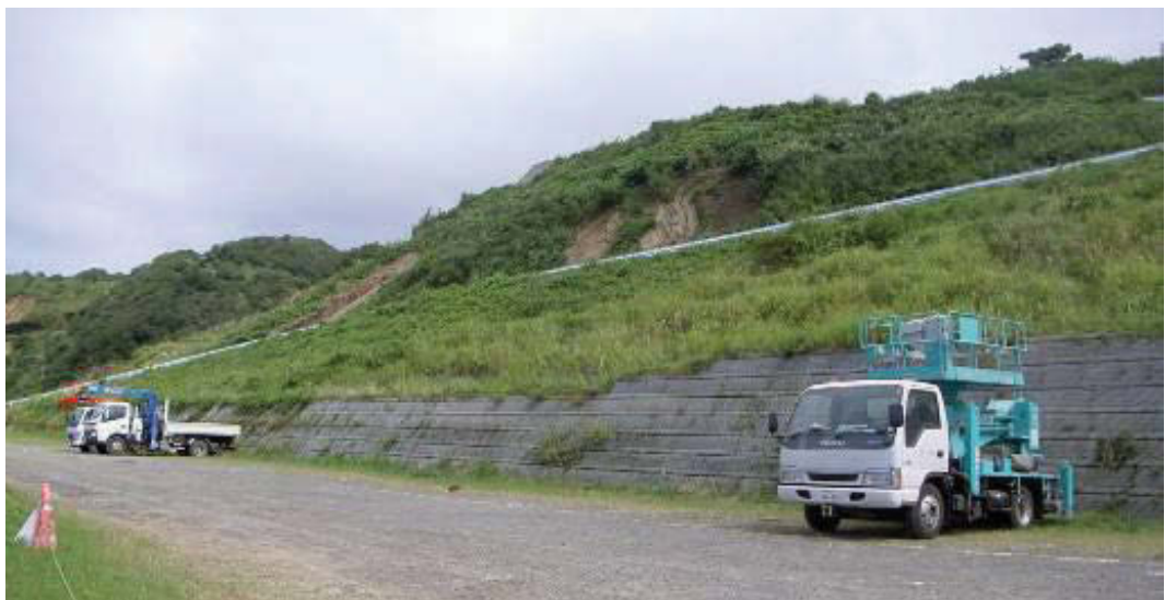
Figure 2.8 RSW with at Agewa with segmental facing panels made of metal mesh (Koseki 2012)
