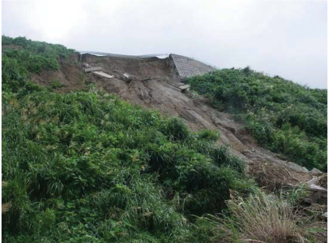
Figure 2.7 Failure of RW for municipal road at Agewa caused by 2007 Niigataken-Chuetsu-Oki earthquake (Koseki 2012)
