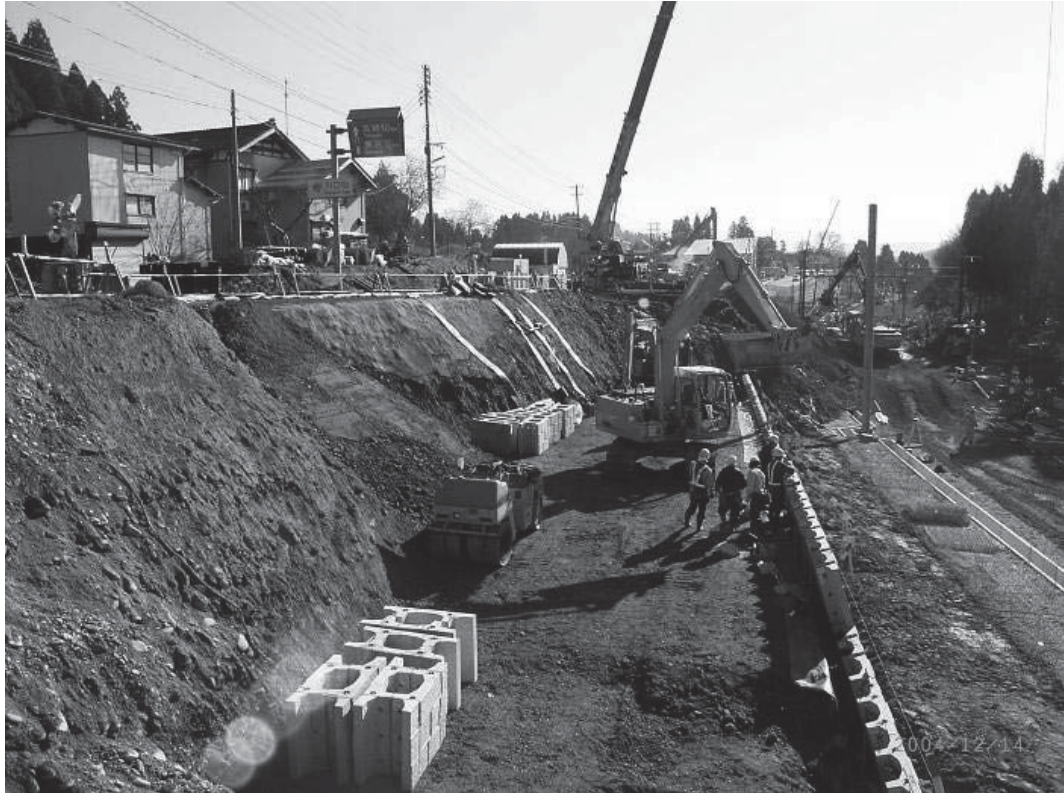
Figure 2.6 Repair of highway embankment as a result of 2004 Chuetsu earthquake (JSCE 2006)
