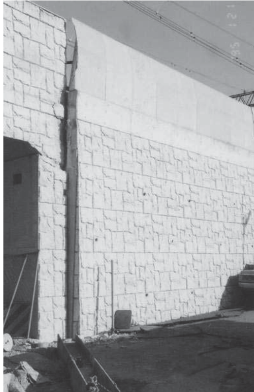
Figure 2.2 Tanata GRS wall after 1995 Kobe earthquake (Tatsuoka, Tateyama & Koseki 1996)
