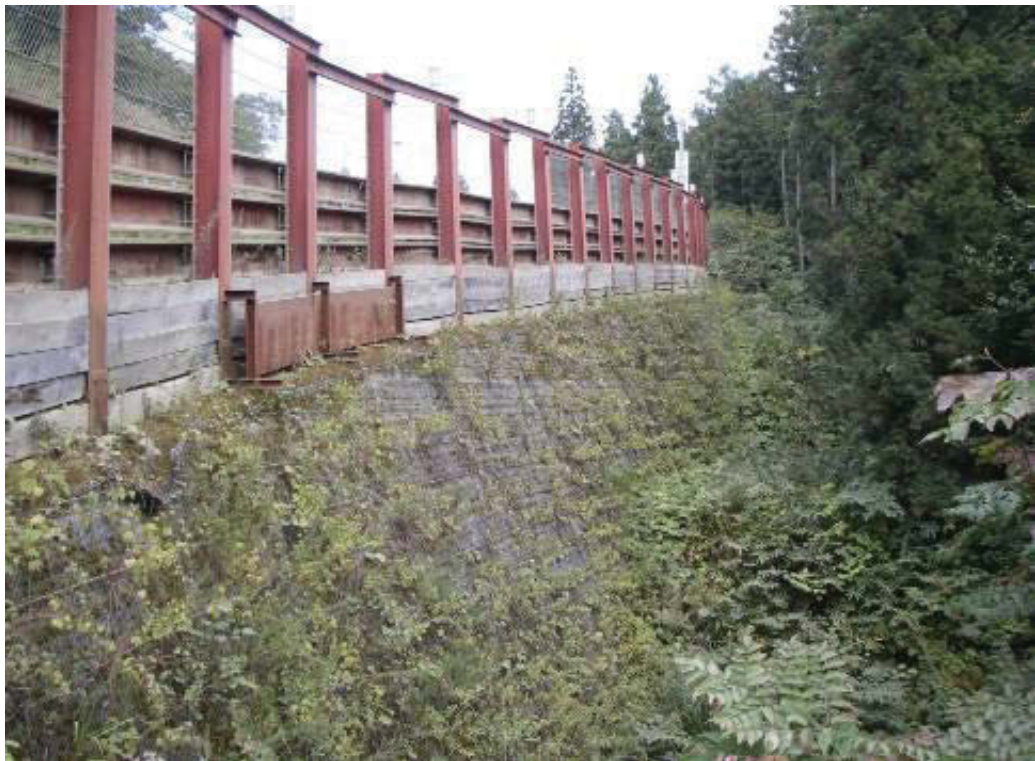
Figure 2.10 RSW with segmented facing panels made of metal mesh at construction site of Isawa dam (Koseki 2012)
