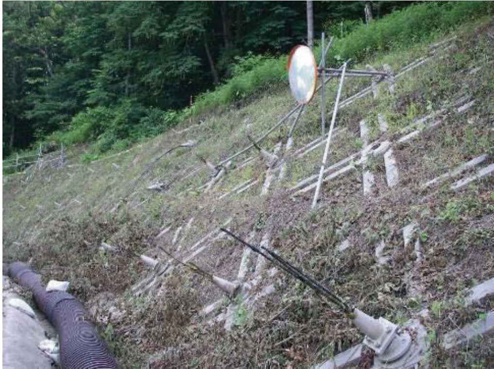
Figure 2.9 Failure of anchor tendons for cut-slope at construction site of Isawa dam caused by 2008 Iwate-Miyagi-Nairiku earthquake (Koseki 2012)
