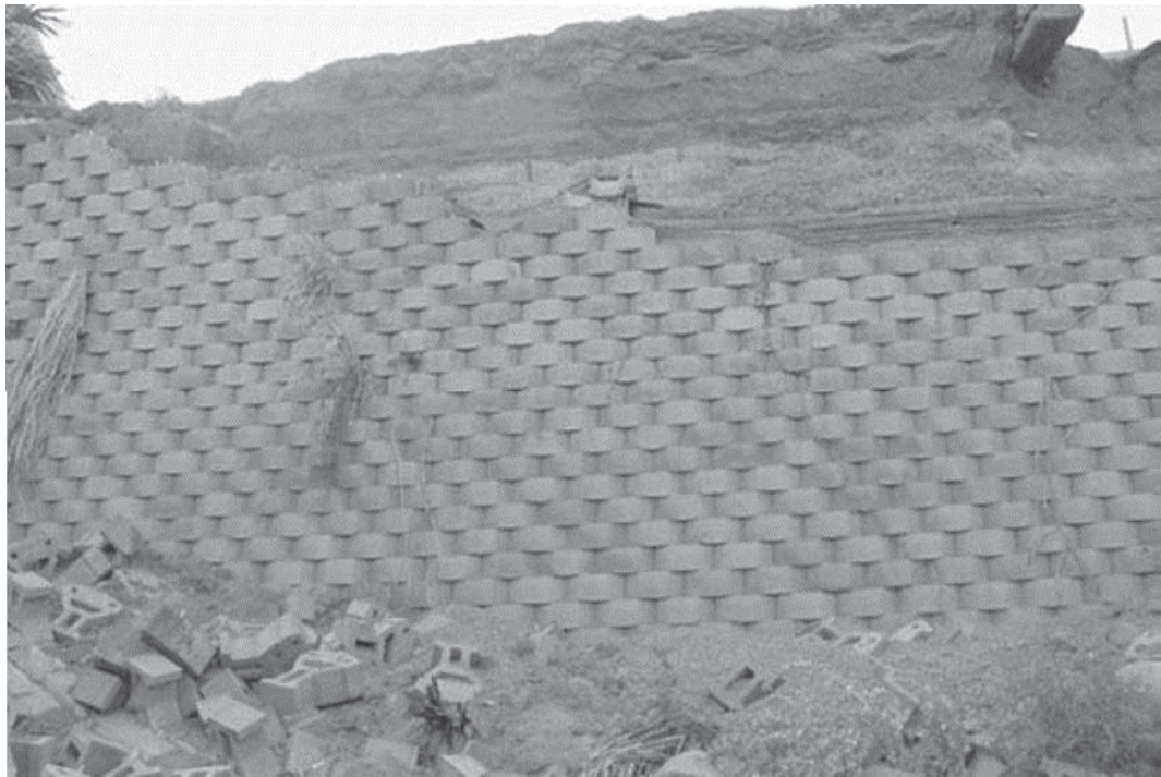
Figure 2.4 Wall failures in El Salvador due to 1.7 m high unreinforced section at top of wall added by the owner after original construction (Koseki et al. 2006)
