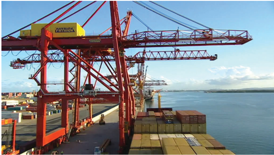
Figure 2-1: Typical QCs employed at the container Terminal in Brisbane, Australia.
