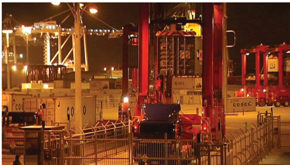
Figure 2-2: ASC servicing a TK in the TIA at the Patrick AutoStrad container terminal located in Brisbane, Australia.
