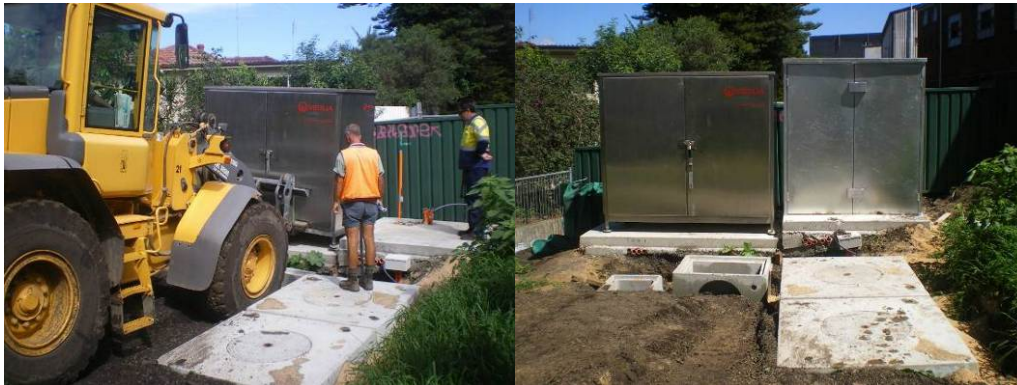
Figure B.6 Delivery and installation of Harvesting Plant cabinets
