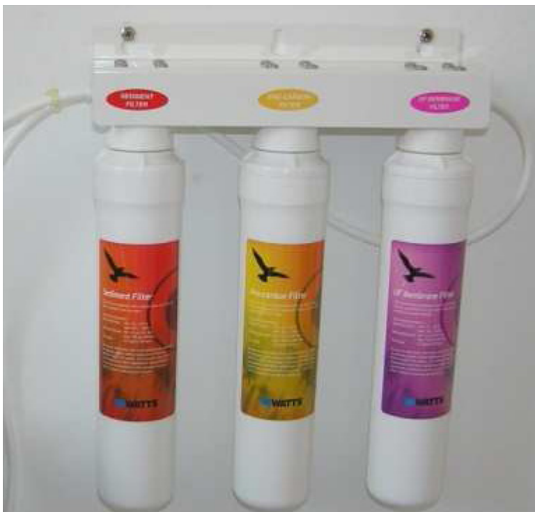
Figure 3.10 Photograph of cartridge filtration system
