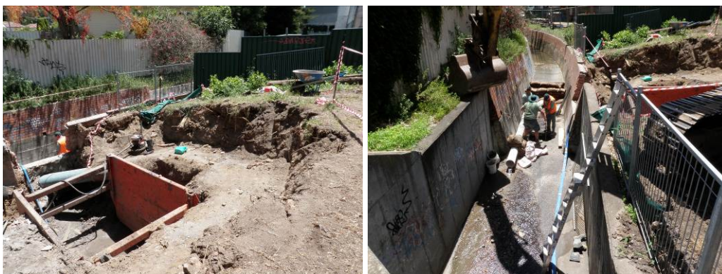
Figure B.2 Excavation of site for sump and pipe installation
