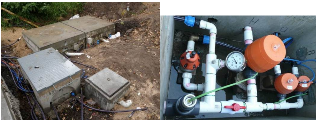
Figure B.7 Completion of control valve pit hydraulics
