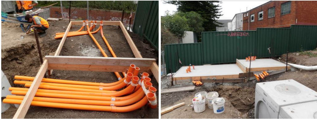
Figure B.3 Installation of conduits for hydraulic line connections through slab
