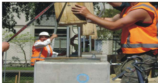
Figure 8.9 Installing frames onto steel rods on concrete plinths
