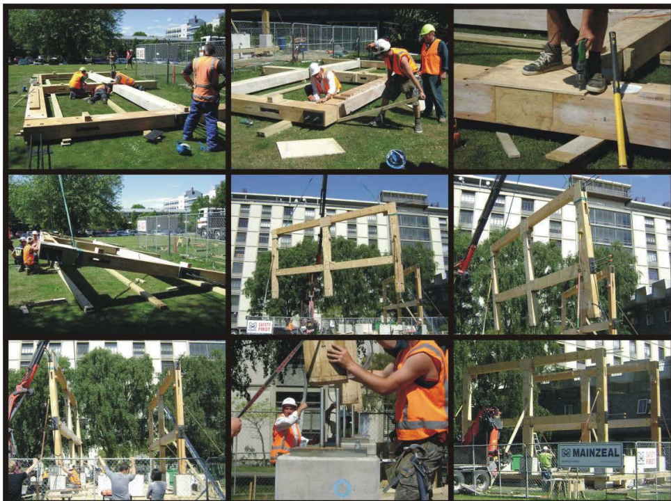
Figure 8.5 STIC office during construction
