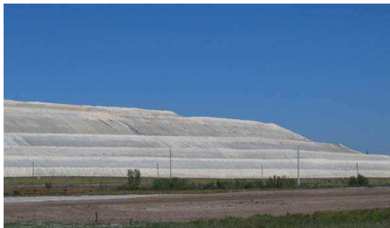
Figure 3. Phosphogypsum stockpile in Florida—byproduct from phosphate fertilizer production often considered too radioactive for reuse (Image from US Environmental Protection Agency).
