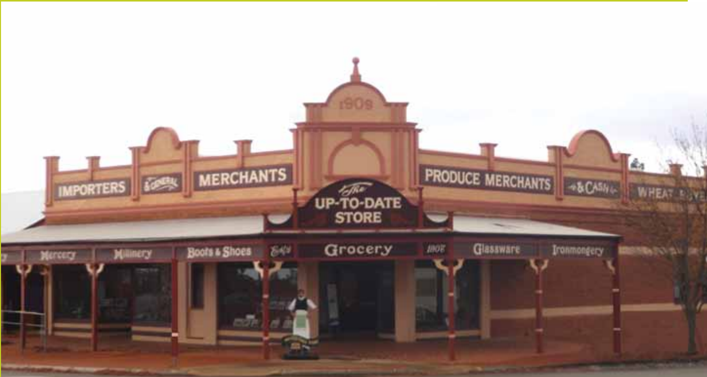
The Up-to-Date Store: as it was originally, and refurbished and renewed, at its centenary in 2009
