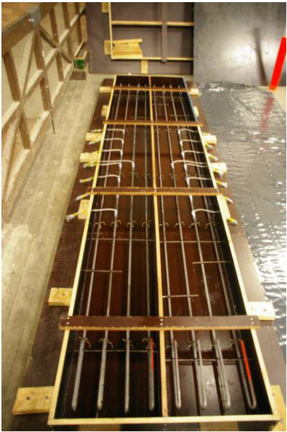
Figure 6.3 General view of slab mould before casting the SCC
