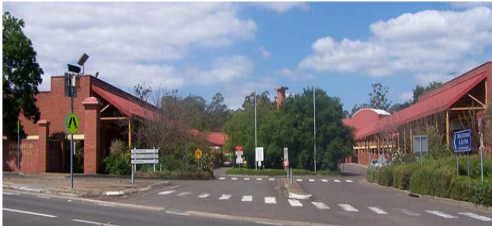
Figure 1: A small level three metropolitan public hospital in NSW
