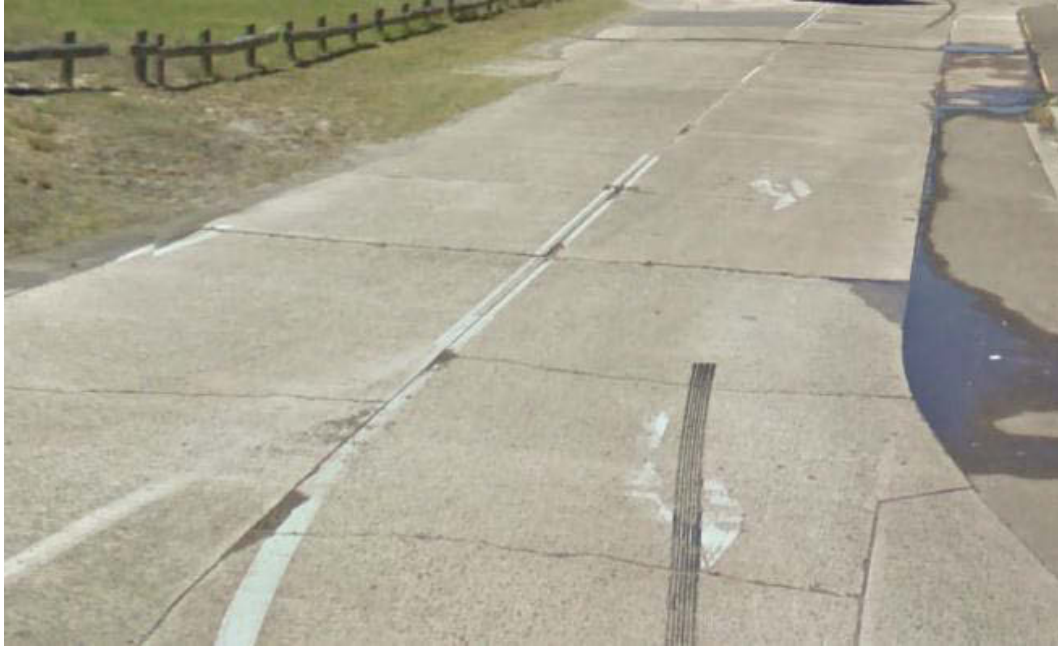
Figure 4.17: Site of concrete survey test, Heffron Park, Maroubra NSW
