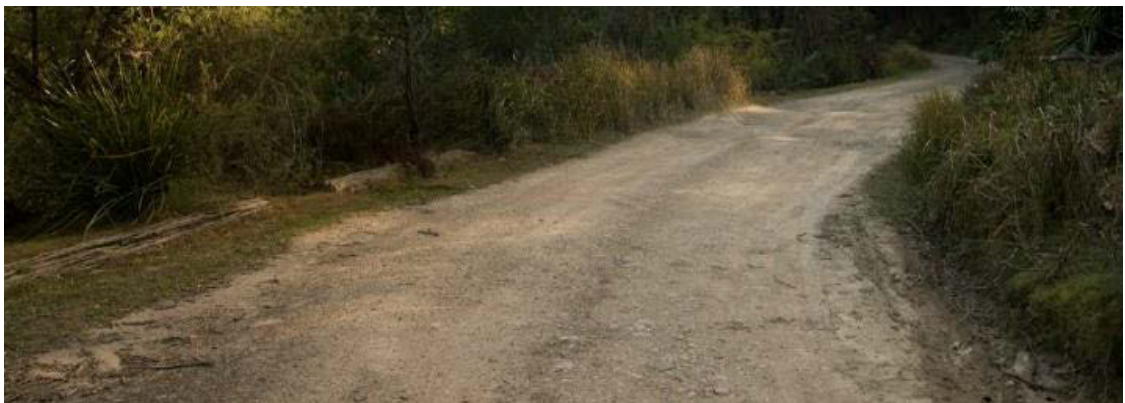
Figure 4.18: Site of gravel survey test, Warumbul Road, Bundeena NSW
