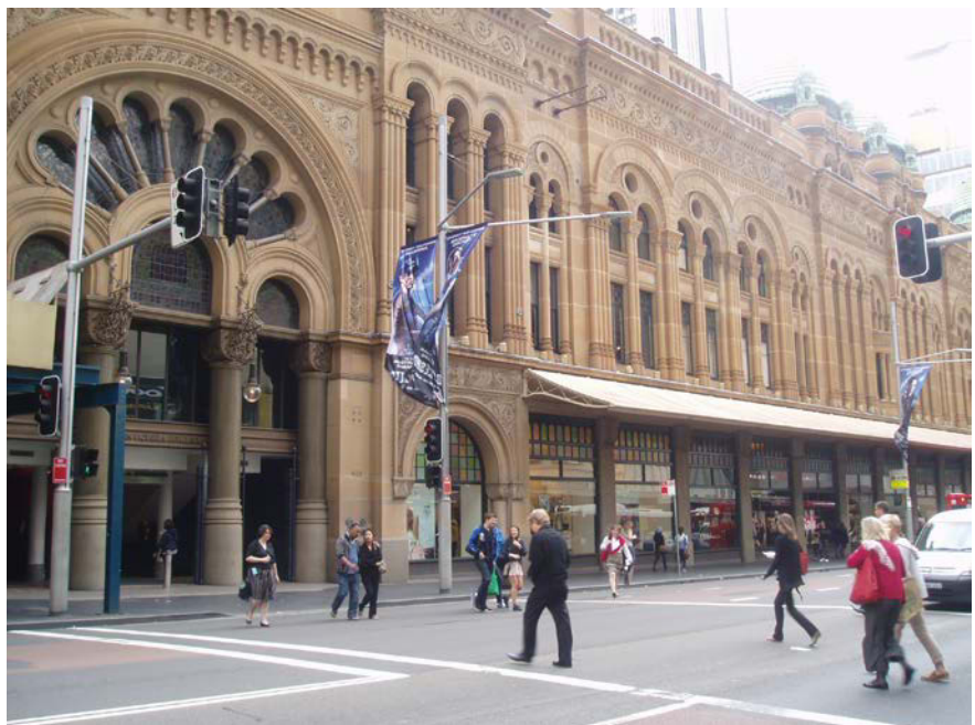
Queen Victoria Building, Sydney CBD Midtown Precinct
