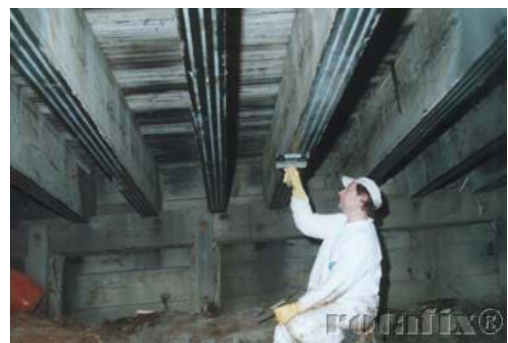
(b) Repairing Timber structure
