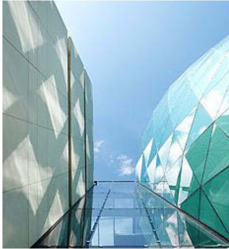
Large glass panel curtain wall
