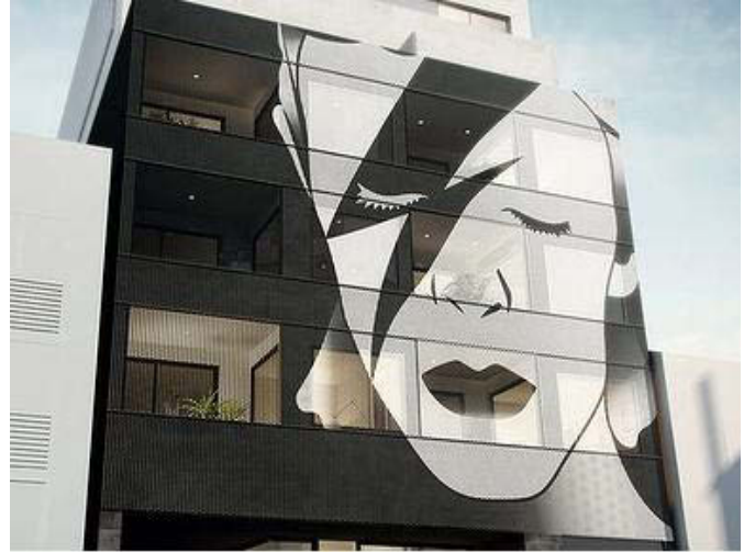
Curtain wall façade with human image
