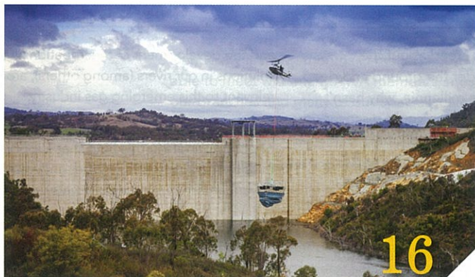
A helicopter lowers a destratification unit into place at Cotter Dam.
