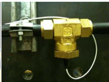
5.4b Pressure Transducer
