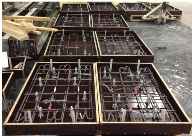
(c) All ten moulds with their located reinforcement mesh
