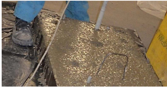
(a) Pouring of concrete
