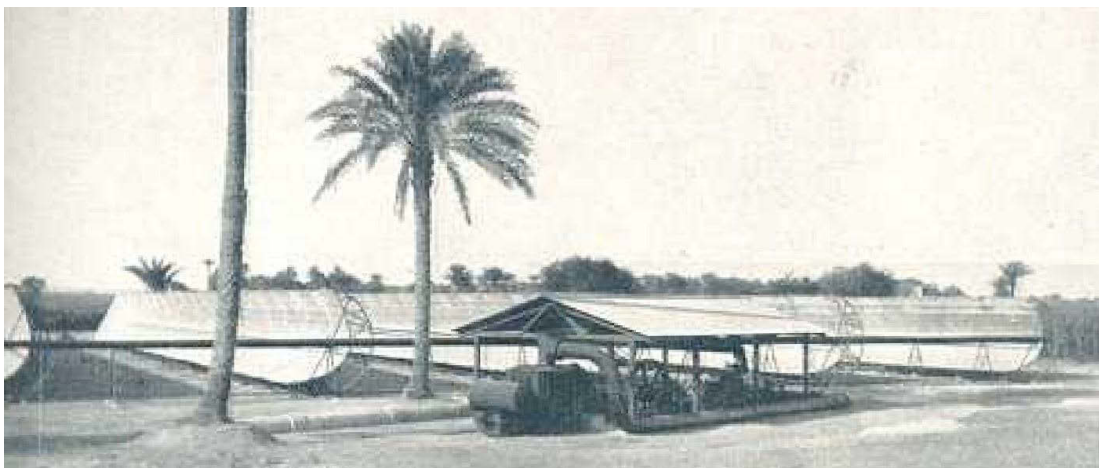
Figure 9: Al Meadi pumping station using the five parabolic troughs with direct steam generation (Stinnesbeck 1914)
