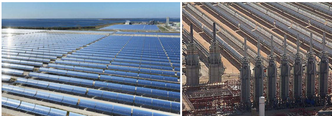
Figure 19: a: 75 MWe equivalent CSP steam boost to Martin Next Generation power station in the USA (Florida Power & Light Company 2010) and b: 100 MWe Shams One plant (Goebel & Luque 2012)
