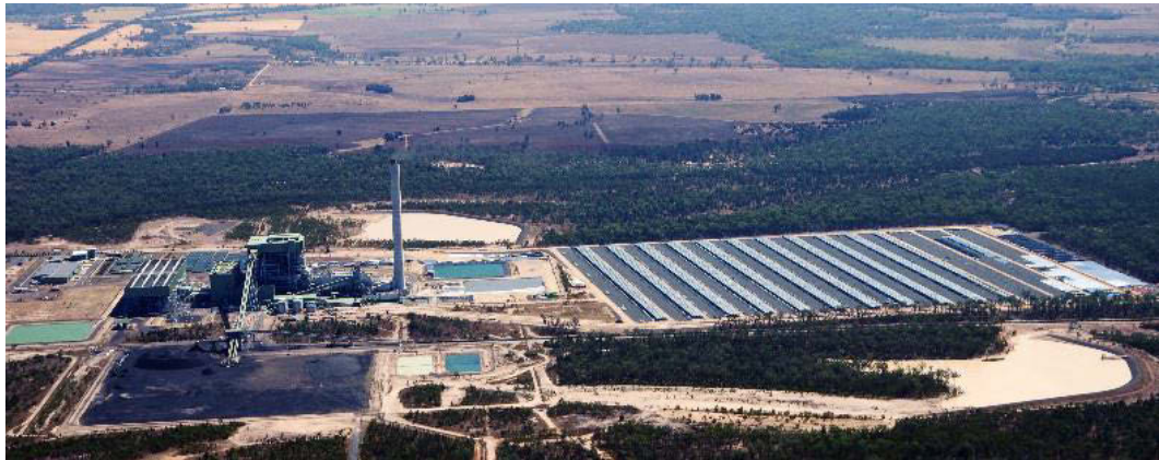
Figure 21: Kogan Creek Solar Boost project under construction as per October 2013 7
