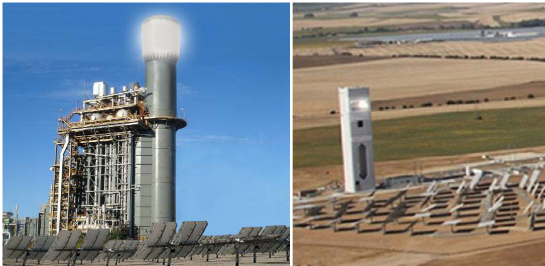
Figure 20: a: 228 MWe solar tower ISCC concept (Peterseim et al. 2012c) and b: 4.6 MWe Solugas tower in Spain (Quero et al. 2013)
