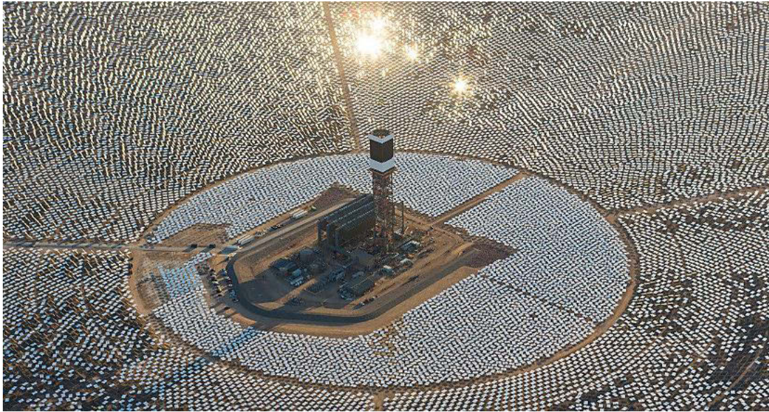
Figure 10: One of three solar tower systems of the 392 MWe Ivanpah power station, USA 3
