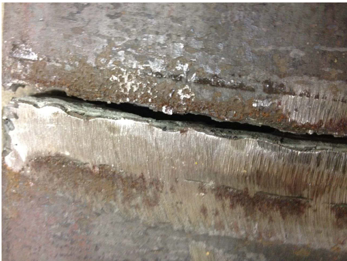
Figure 4-11: Fully developed fatigue crack along the weld toe in a ground flush specimen
