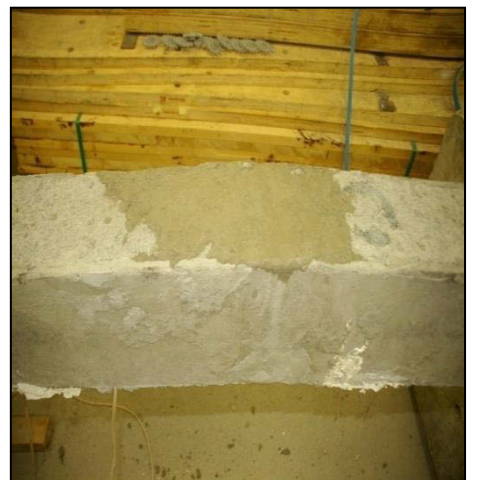
(d) Gaps filled in after exposing the concrete substrate
