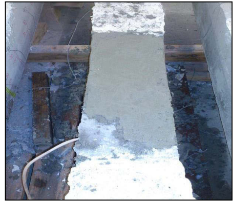
(b) Gaps filled with repair mortar
