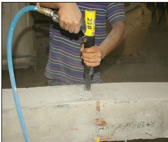
(c) Exposing the concrete substrate
