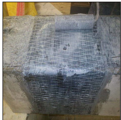
(f) applying pressure with a roller
