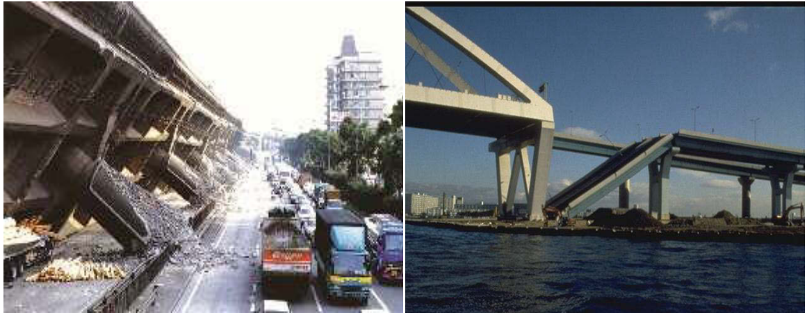
Figure 1.1. Kobe earthquake, 1995, Japan
