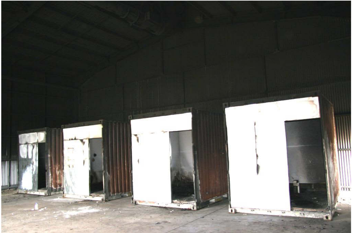
Figure 4.1: Warehouse within QCESA facility housing four shipping containers (burn cells).
