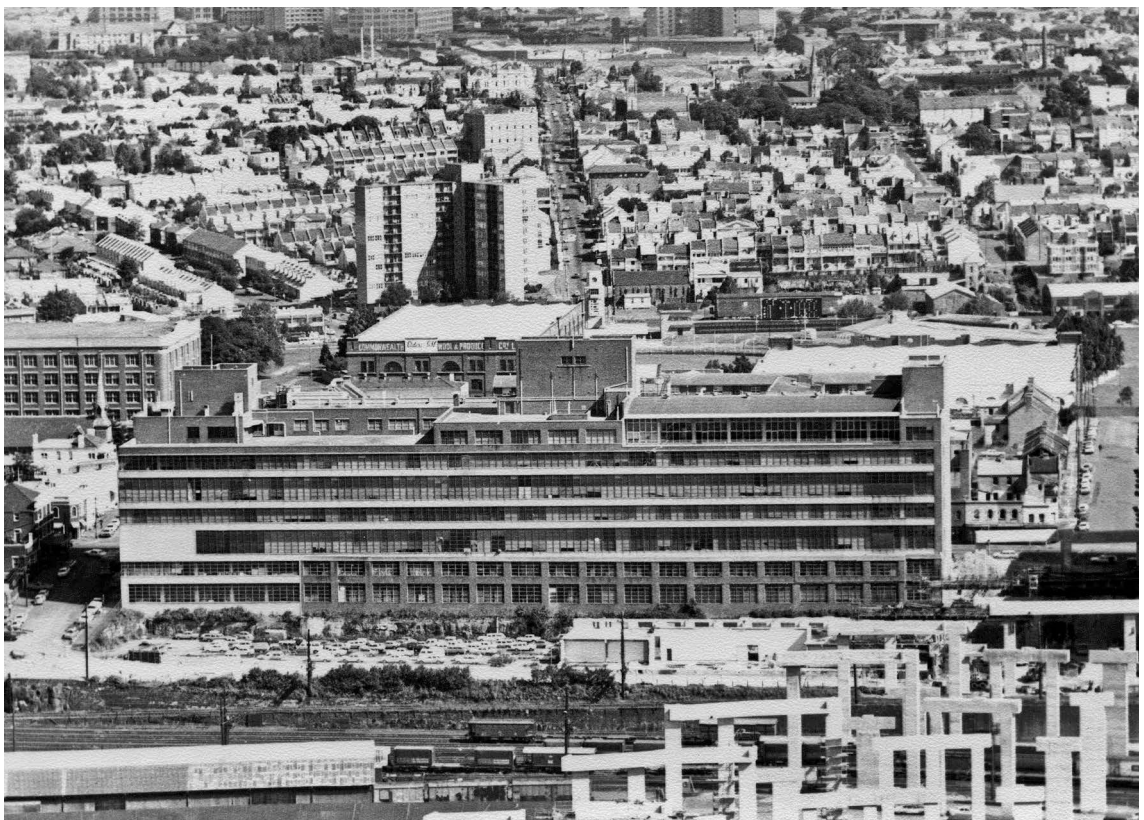
Fig. 12 View south-west to the rear side of the NSW Government Printing Office, Ultimo, early 1980s, showing the Eastern Distributor under construction in Darling Harbour. Courtesy the City of Sydney Archives, Sydney Reference Collection. File #039/039781, citation SRC13384. Reproduced with permission.
