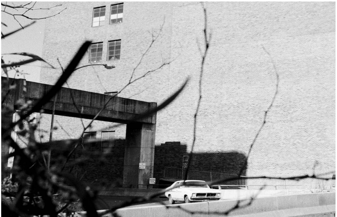
Figs 40–41 Exterior (and detail) of the Government Printing Office building, 1985, looking south down Harris Street, Ultimo, showing the ramp and the 'For mad men only' graffiti. Copyright of the Crown, reproduced with permission, courtesy of the Mitchell Library, State Library of New South Wales, Sydney. SLNSW call no. Government Printing Office 4 – 40363. In Fig. 41 the spray-painted door is faintly visible above the vehicle.
