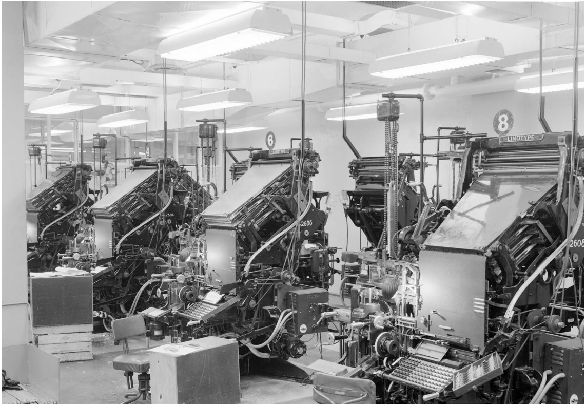
Fig. 68 The Linotype Room at the new Government Printing Office, 1959. Many of these machines remained in use at the Government Printing Office well into the mid-1980s. Courtesy of the Mitchell Library, State Library of New South Wales, Sydney. SLNSW call no. Government Printing Office 2 – 13671.
