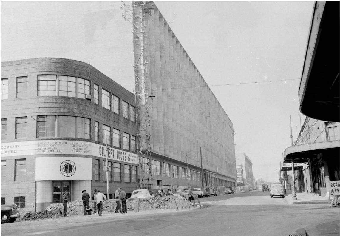
Fig. 6 The new Government Printing Office building, under construction, 1957, Harris Street, Ultimo, looking south. Courtesy of the Mitchell Library, State Library of New South Wales, Sydney. SLNSW call no. Government Printing Office 2 – 08781.
