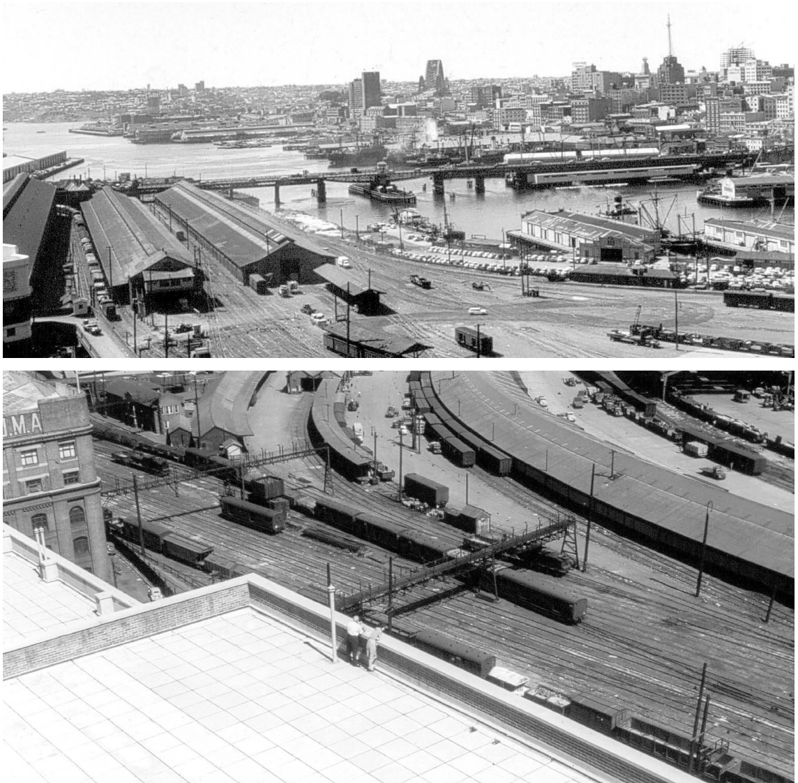
Figs 9–10 Two views from the lift overrun at the top of the NSW Government Printing Office building, down to the flat part of the roof and the Darling Harbour Railway Goods Yard, c. 1960s. Photographs by John Cusack, reproduced with permission.
