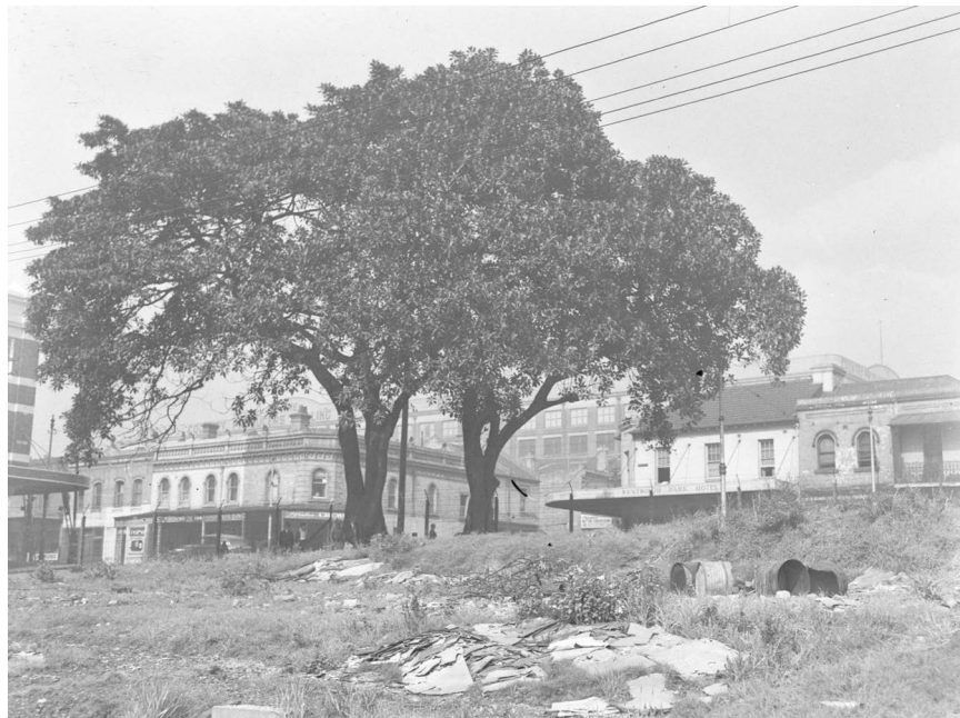
Fig. 32 Site of the new Government Printing Office, Ultimo, 1950, before the removal of the fig trees. Courtesy of the Mitchell Library, State Library of New South Wales, Sydney. SLNSW call no. Government Printing Office 1 – 07729.
