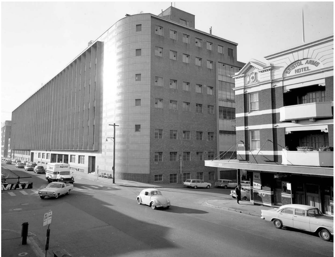
Fig. 26 NSW Government Printing Office, Harris Street, Ultimo, 1967. Copyright of the Crown, reproduced with permission, courtesy of the Mitchell Library, State Library of New South Wales, Sydney. SLNSW call no. Government Printing Office 2 – 37773. With thanks to Mark O'Brien, Global Switch Sydney.
