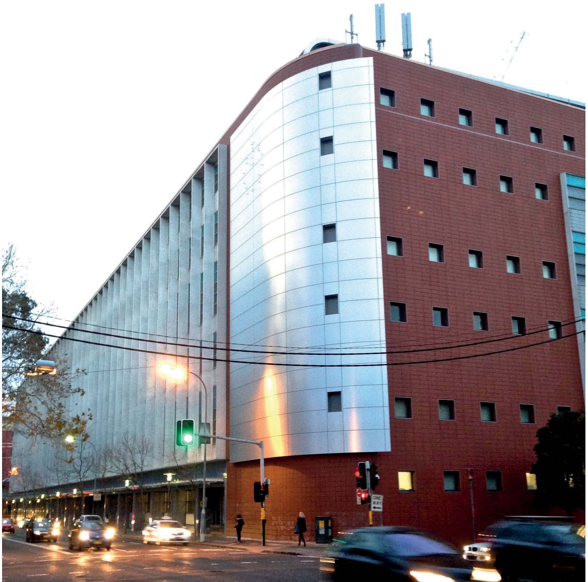
Fig. 47 The former Government Printing Office building in Ultimo, Sydney, 2013. Now extensively refurbished and occupied by the data-storage company Global Switch. Photograph by the author.
