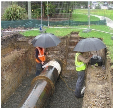
Fig. 7. Obtaining testing data (BEM scanning being done on the test bed).
