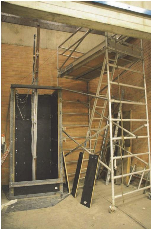
a) Scaffold to build the frame
