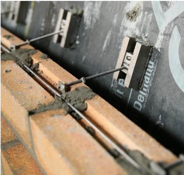
Figure 21: Small temporary restraint nut supporting sloping in brickwork
