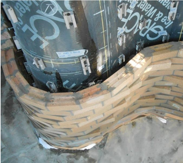
Figure 6: Plan curvature of brickwork requiring regular brick cutting
