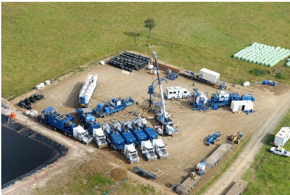
Figure 9 CSG well being fracked at Gloucester gas project (NSW)
