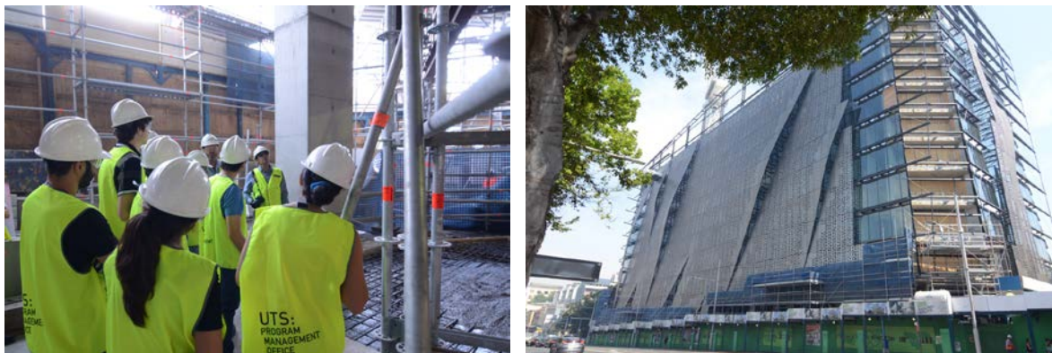
Figure 2: Visit to the UTS new engineering and IT building construction site
