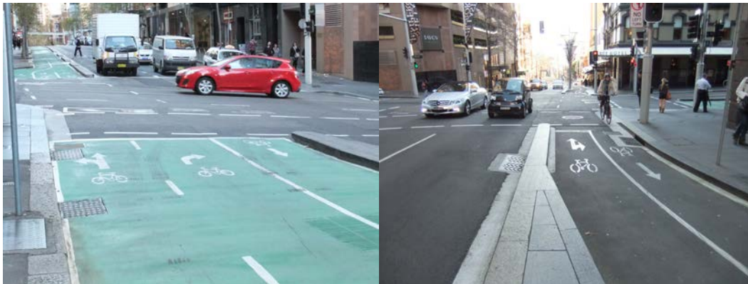
Figure 2: Kent St facing south towards King St (left) King St facing west toward Kent St (right).
