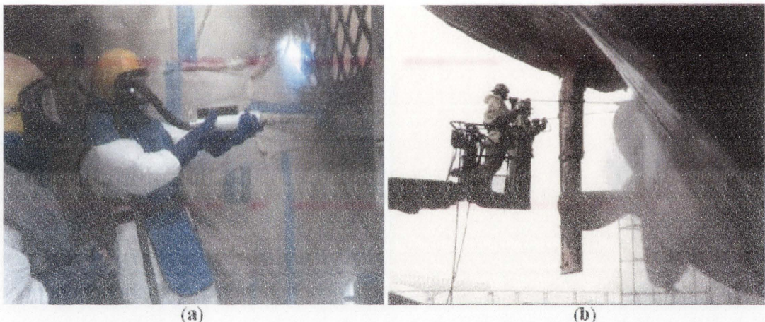
Figure 1.1 Examples of industrial applications in which operators can be replaced by a mobile robot manipulator to interact with complex environments in hazardous workplaces: (a) Sandblasting operation in steel bridge maintenance, (b) Vessel maintenance (from Broadbent's, Inc)
