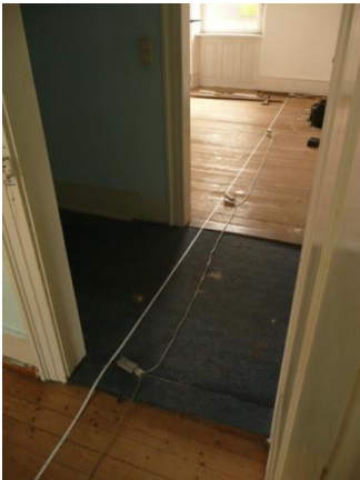
Figure 12 Investigation of beam without opening the floor
