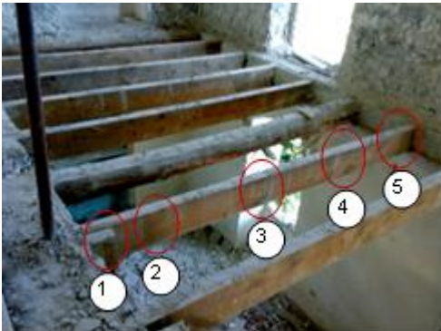
Figure 6 Typical example for stress wave-based condition assessment in structural timber
