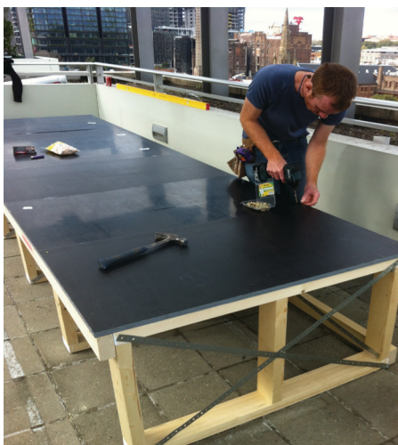
Plate 2 Gumal under construction.
