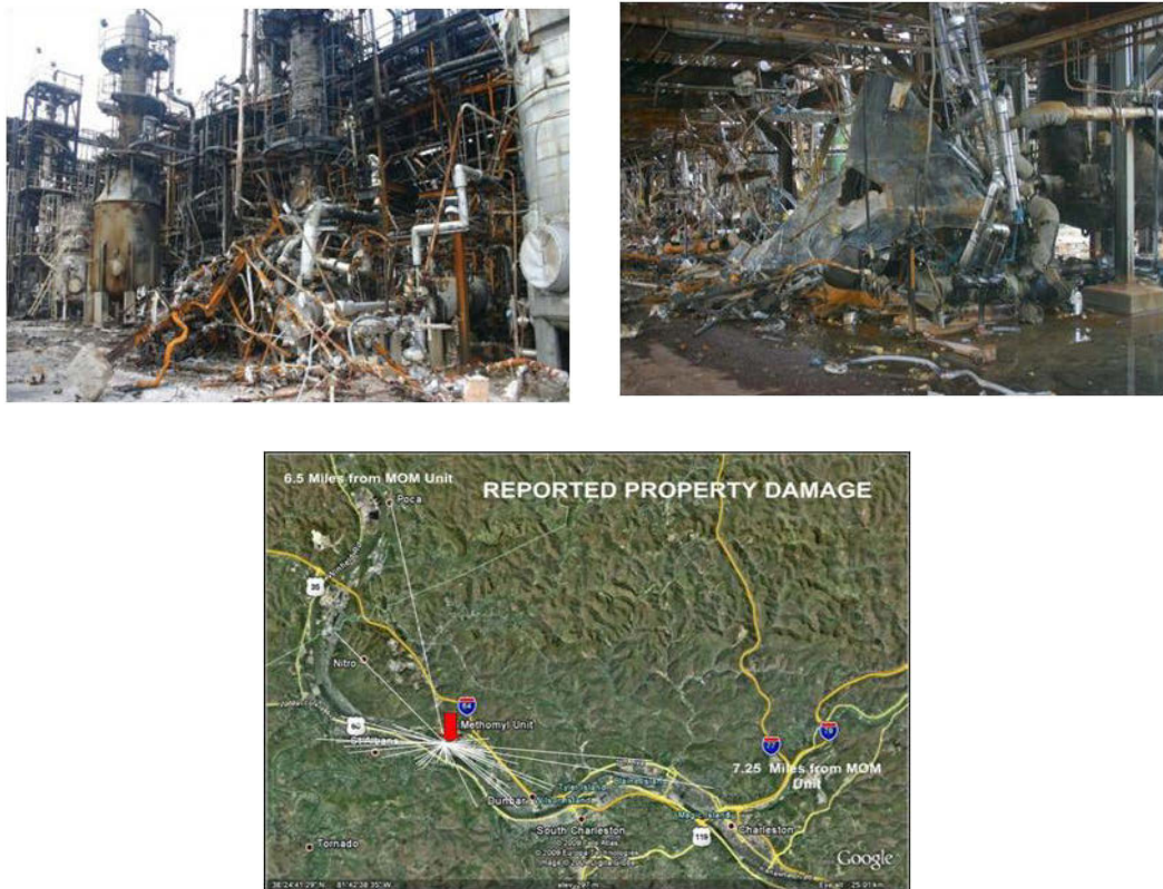
Figure 3.1: Methomyl facility damage and aerial view of reported damaged properties
