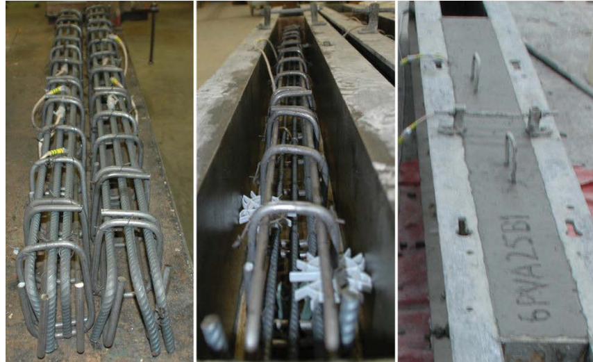
Figure 22. Preparation of concrete beams
