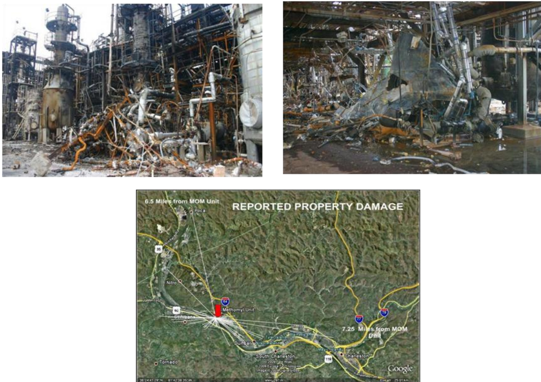
Figure 1: Facility damage and aerial view of reported damaged properties (CSB, 2011).
