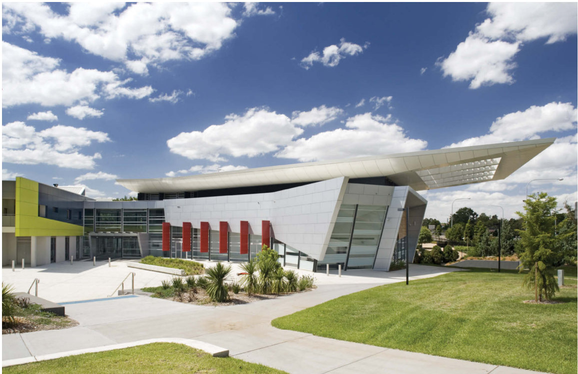
Figure 1: Campbelltown Arts Centre, photo, 2005, Campbelltown City Council.
